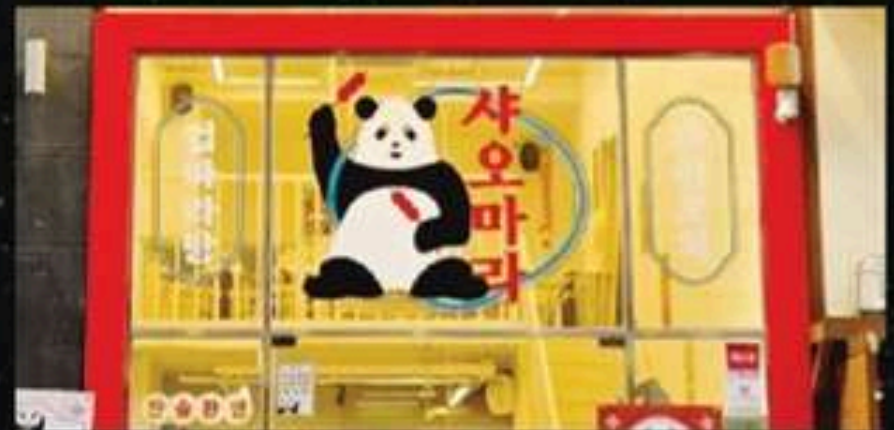
Exterior Vinyl Wrapping (construction)
